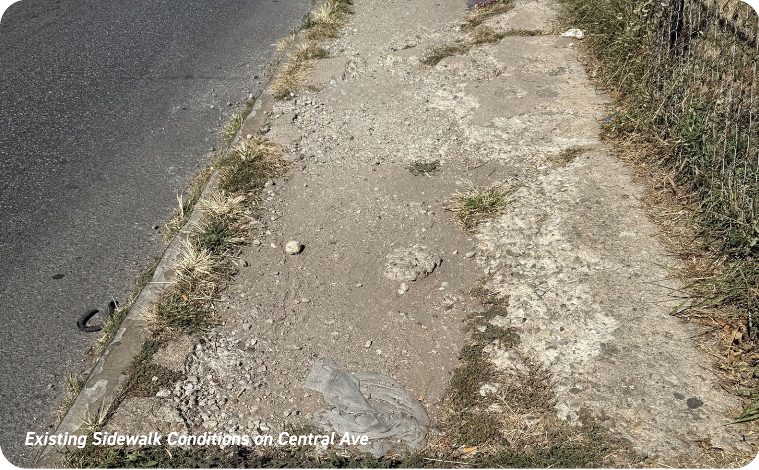
Existing Sidewalk Conditions on Central Ave
