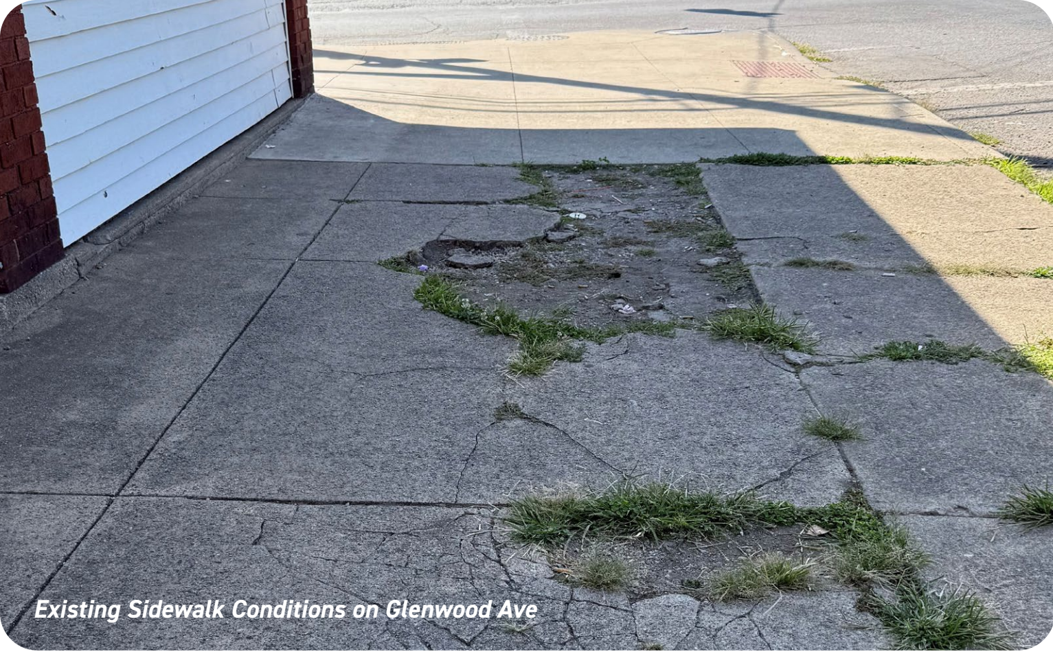
Existing Sidewalk Conditions on Glenwood Ave
