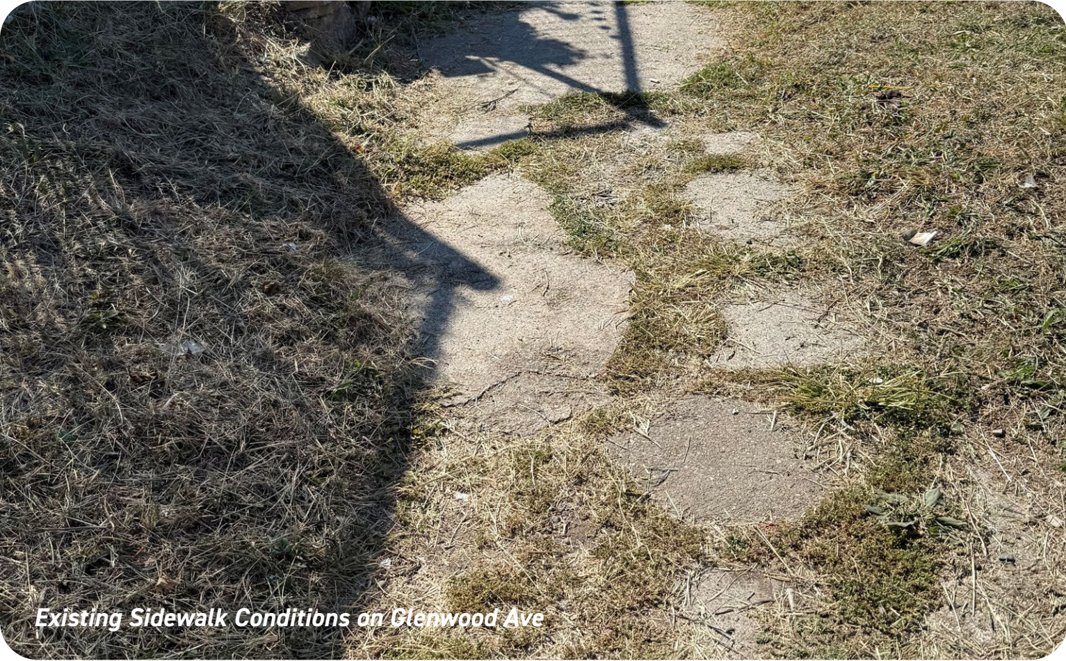
Existing Sidewalk Conditions on Glenwood Ave
